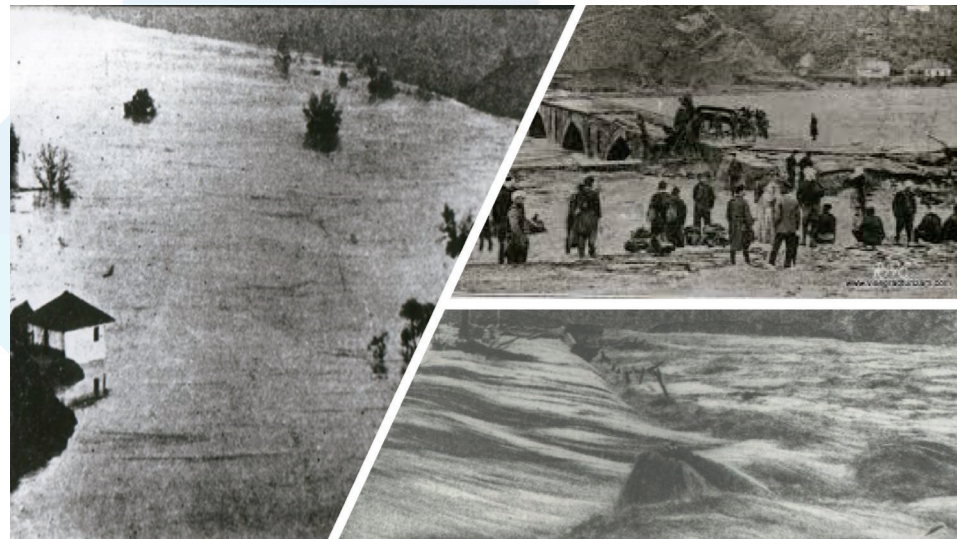
The 1896 Drina flood in Višegrad. Recorded water level of the Drina was 1m over fence on the famous bridge of Mehmed Paša Sokolović in Višegrad. The entire Podrinje was affected by this flood.
